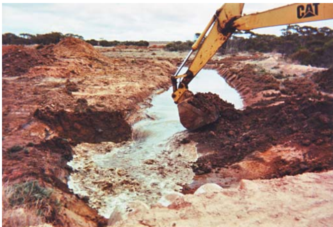
Groundwater fills the drain during construction.
