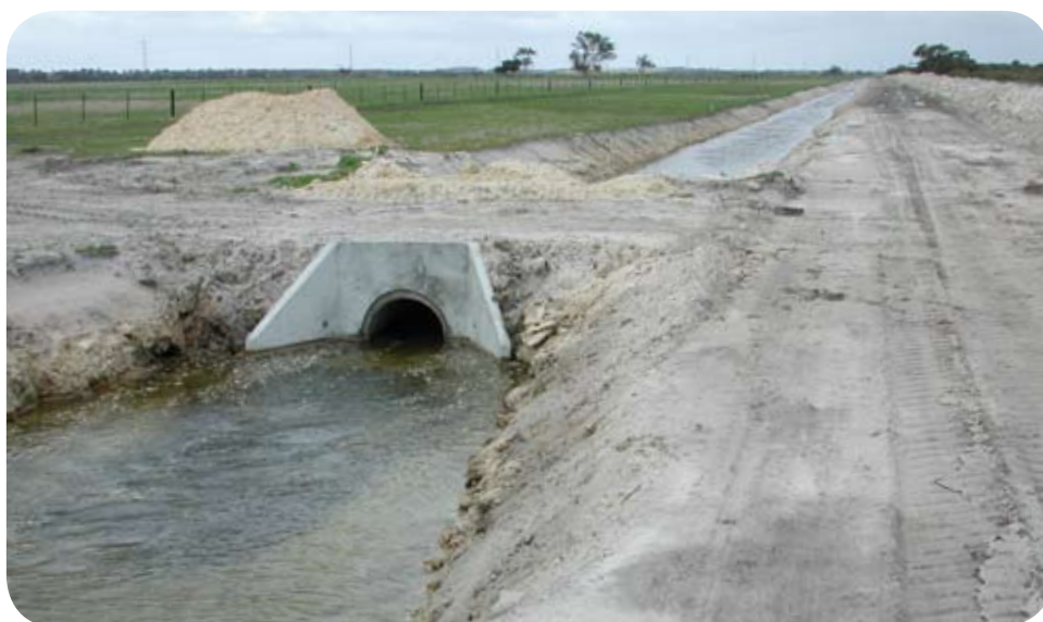
Deep drains can effectively remove excessive run-off and reduce waterlogging but are relatively expensive to construct
